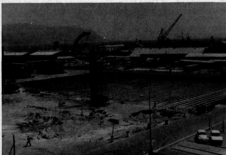
Simonstown Synchronlift and rails to move submarines
