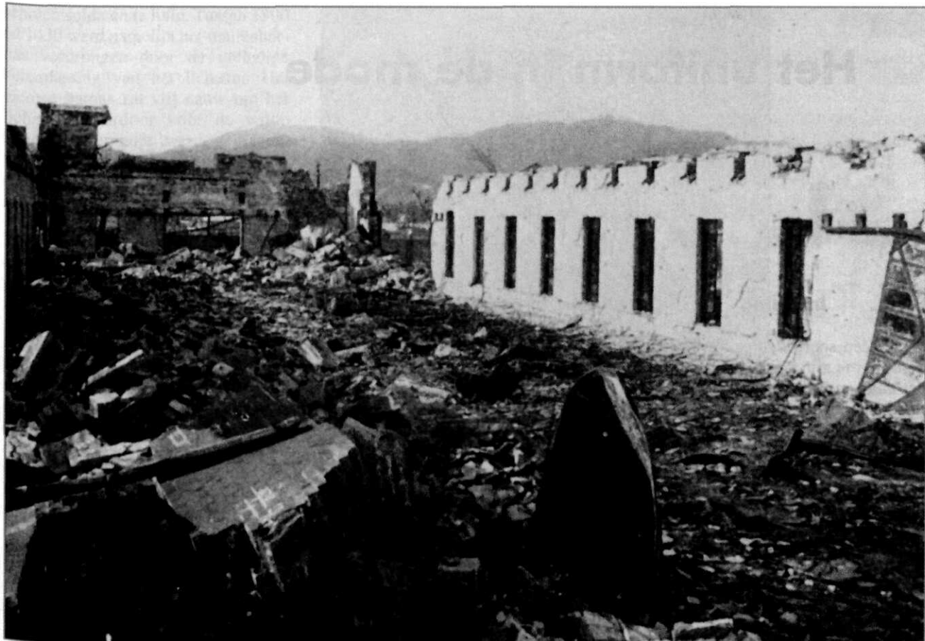
Afb. 3 The remains of a barrack at the Japanese Army Divisional Grounds, 4,200 feet from ground zero at Hiroshima (Bron: The United States Strategic Bombing Survey, Washington 1994)
