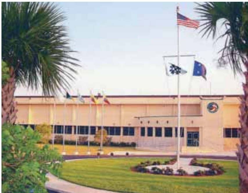
Hoofdkwartier JIATF-South te Key West, Florida (Foto JIATF-South)
