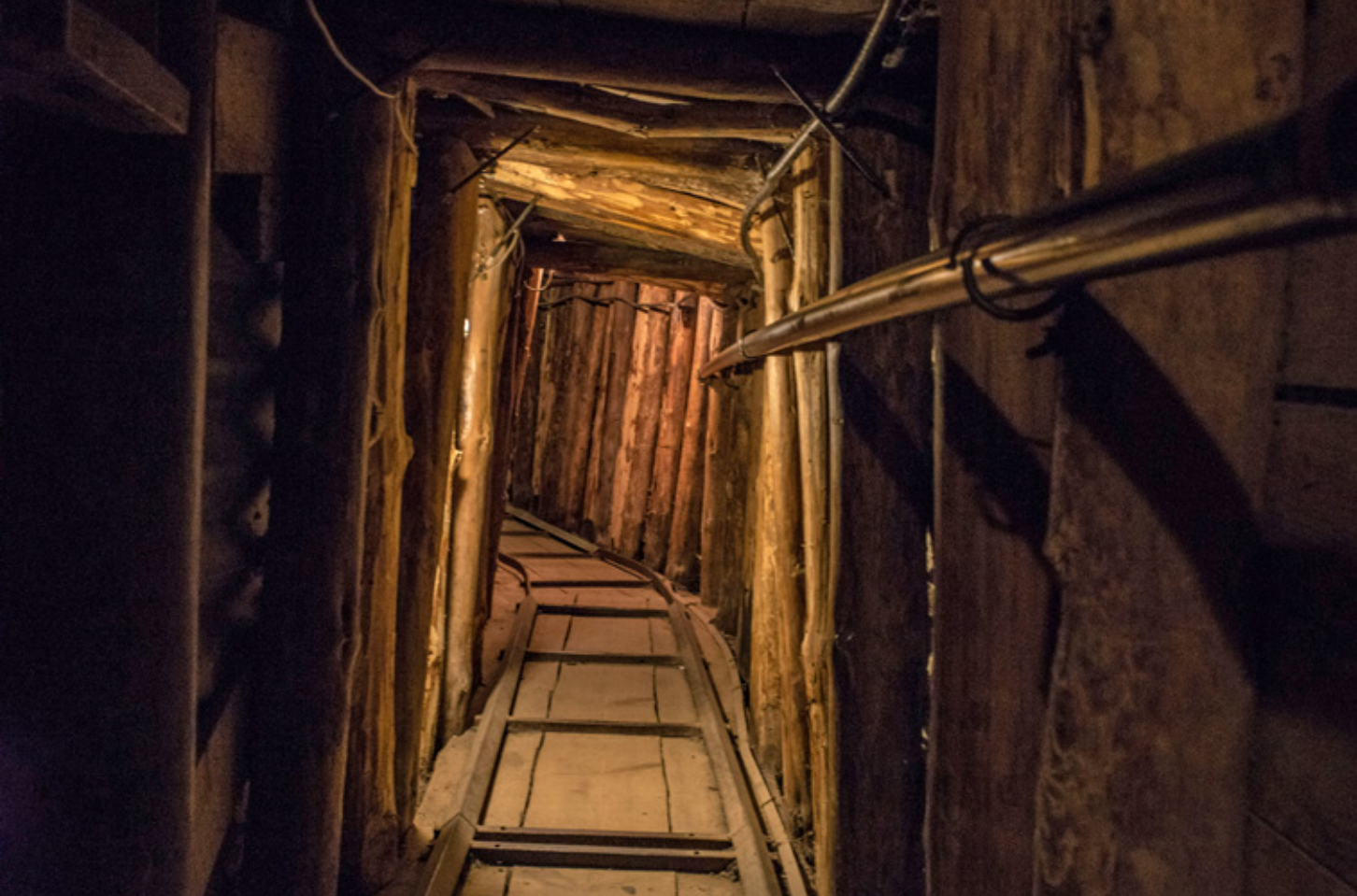
The tunnel near the Sarajevo airport
